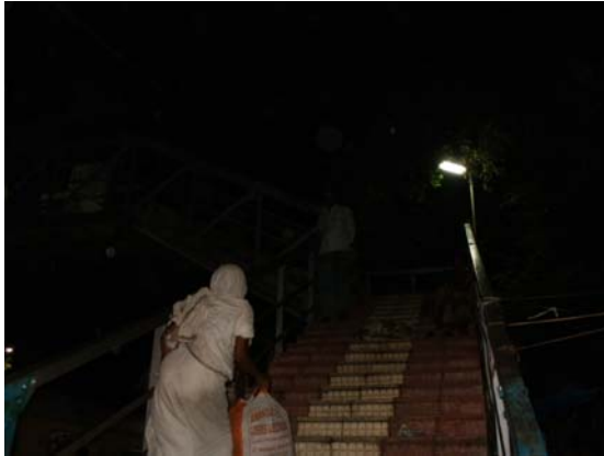
Poorly lit over-bridge
