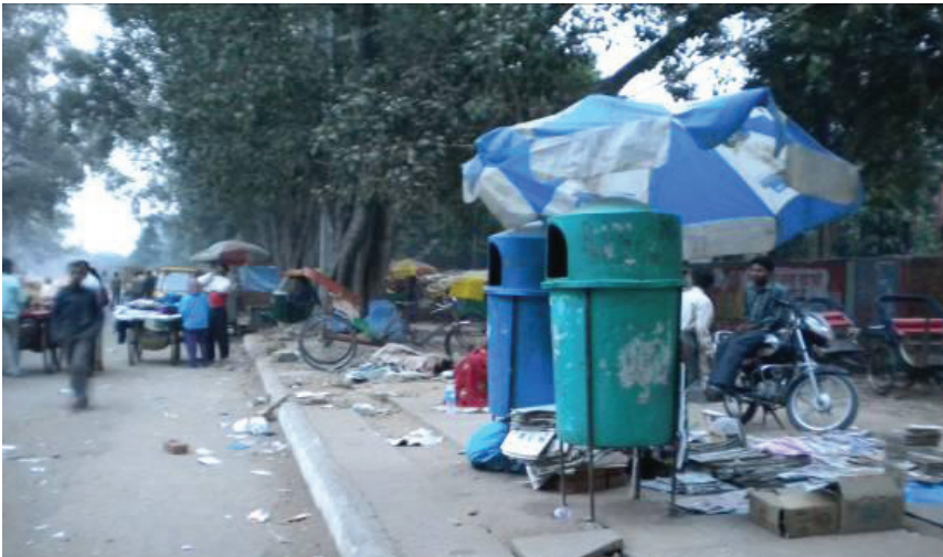
Condition of pavement in Ajmeri gate
