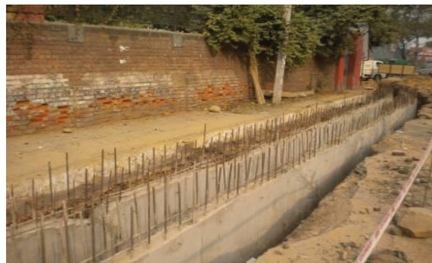
Under construction site along the busy lane towards Kamla Nagar Market in University of Delhi (North Campus)
