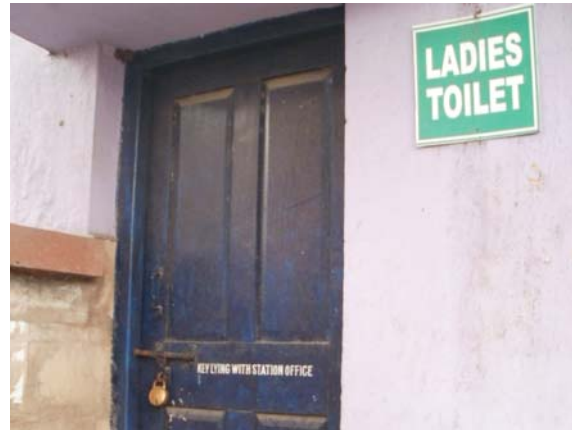
Locked ladies toilet, signage in English only
