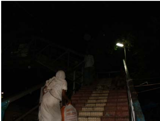
Poorly lit over-bridge
